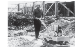
First reversible vibratory plate by Wacker
